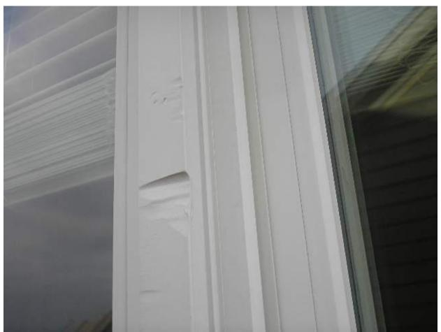
14.15. Some exterior trim has raised nail bumps and rough edges, like trim around overhead garage door. Trim appears to be a type of hardboard man-made trim here.
